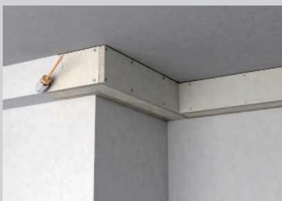
Closing surface treatment through painting or papering.
