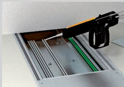
Application of the fire protection foam directly under the wall.
