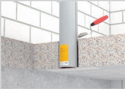
With ceiling mounting, use a lined body to prevent the pipe shell from falling out.
