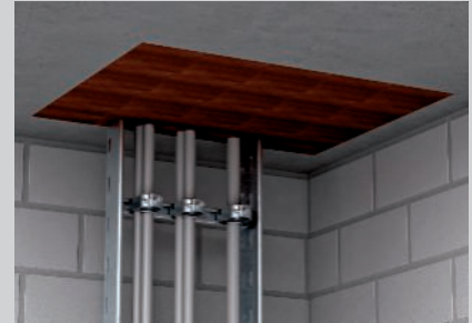
Tight-fitting installation of the blocks in the ceiling penetration.
