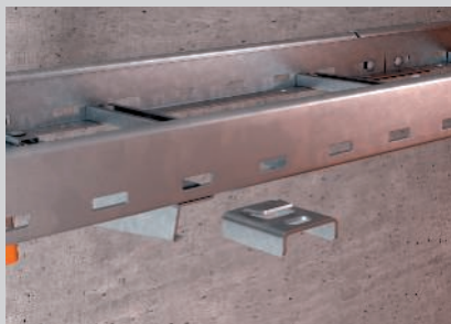
Attachment of the connection component on the lower flange of the ladder rail.
